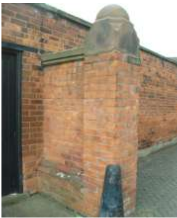
Brick wall at threshold to the Cobbles
