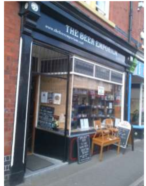
A traditional shop front in the Conservation area
