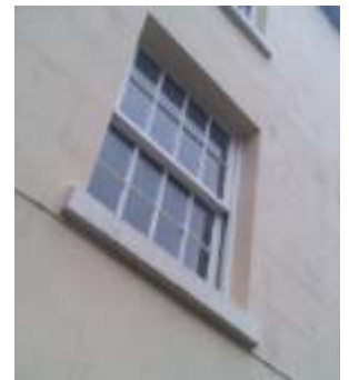
8 over 8 sash window
