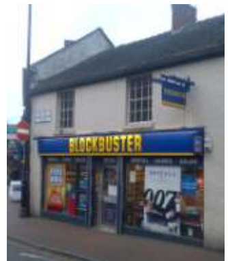
Poor shop fronts and public realm detract from High Street/High Town
