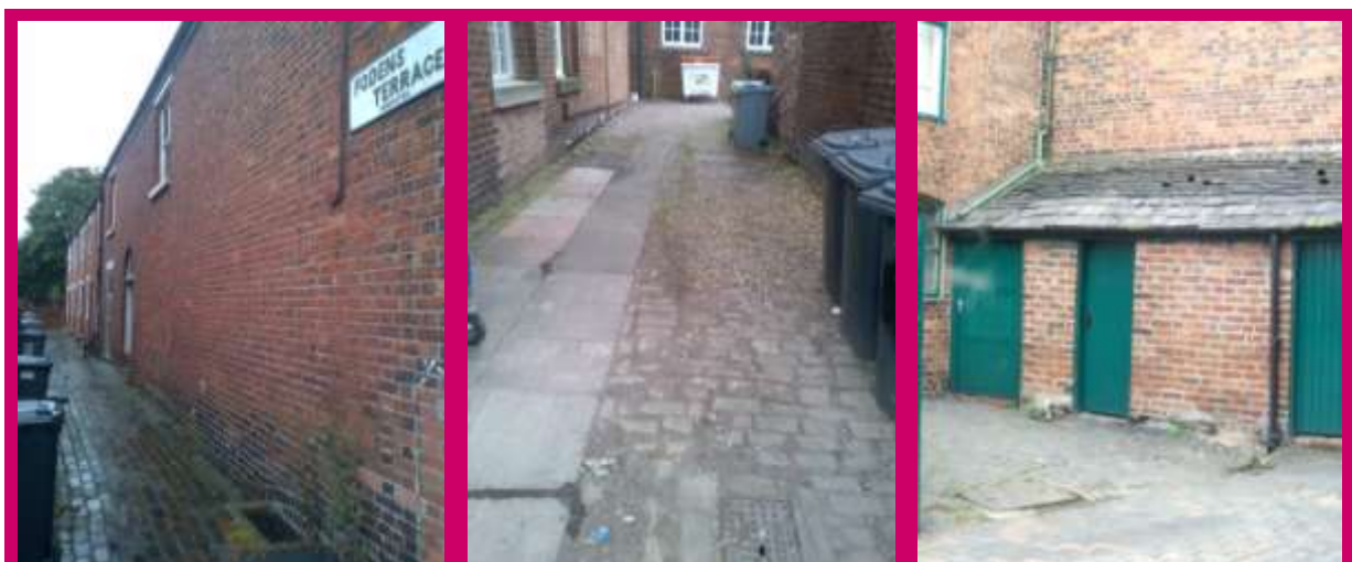
Remnant traditional paving materials: stone sets and Staffordshire blue brick paving within the area
