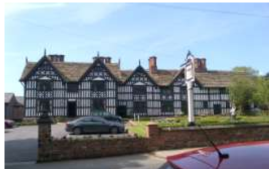
Old Hall – grade I timber framed building
