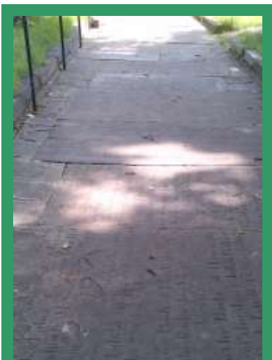
The pathways leading up to St Mary's Church from High Street and Crown Bank create a unique public realm. The stone flags include re-used grave stones. The inscriptions create texture and character
