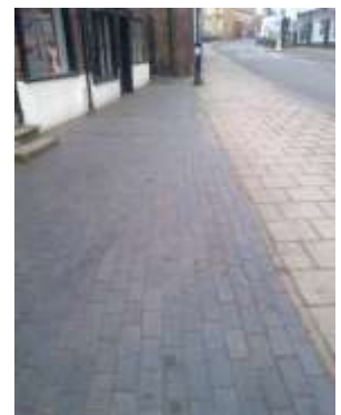
Intersection of old and new surfaces in Crown Bank and High Street. Poor intersection in crown Bank with loose edge of tarmac overlying cobble street
