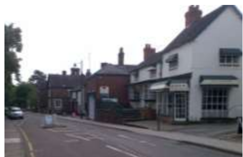
Inappropriate alterations to 45 High Street
