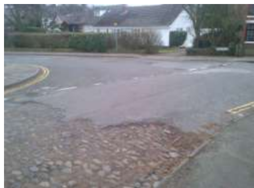
Intersection of old and new surfaces in Crown Bank and High Street. Poor intersection in crown Bank with loose edge of tarmac overlying cobble street
