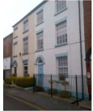
6 – 8 Hope Street with painted brickwork
