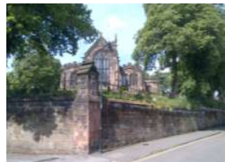
Artificially elevated church site and Sandstone wall
