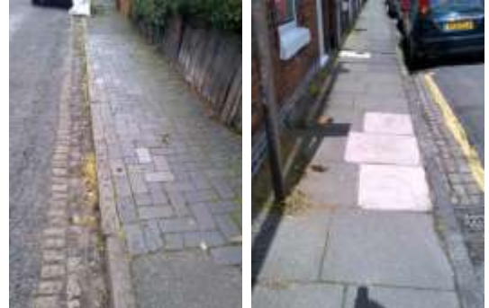
Some historic materials but most pavements are in concrete slabs or tarmac that detract from the area
