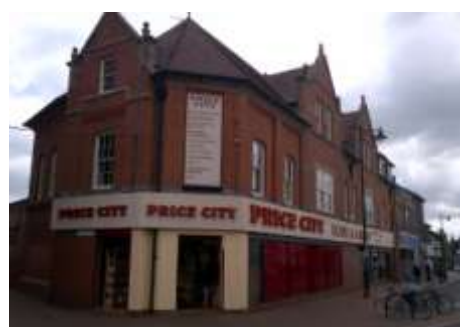
Brick is the predominant facing material
